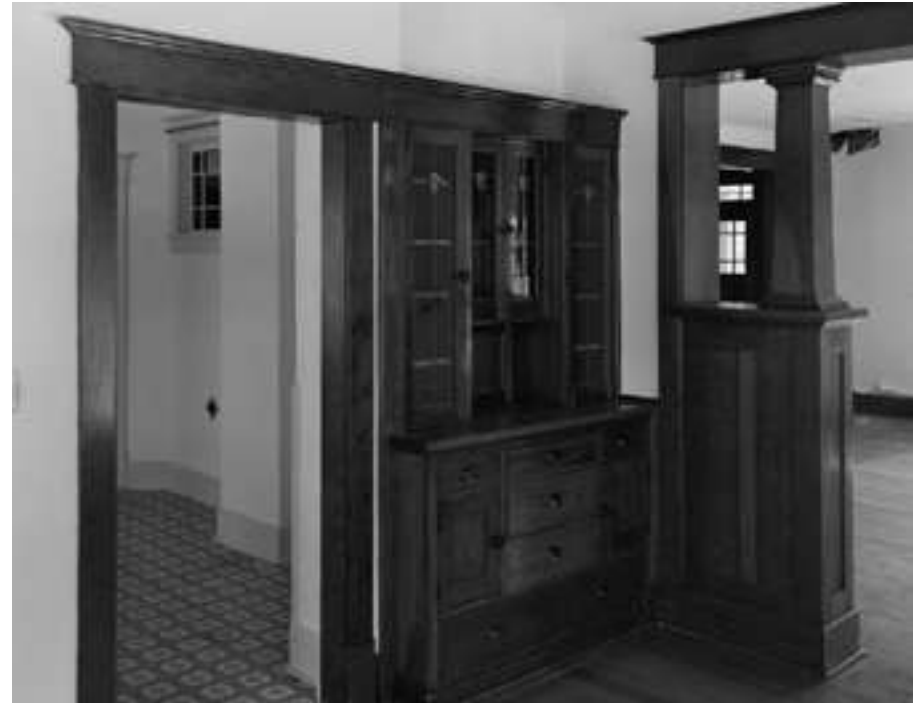
Power Foreman's Bungalow, Thompson Falls, Sanders County, Montana
