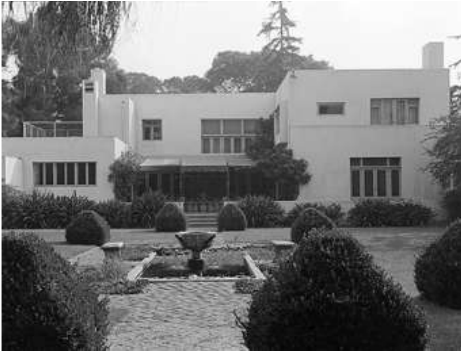
Walter Dodge House, West Hollywood District, Los Angeles, Los Angeles County, California
