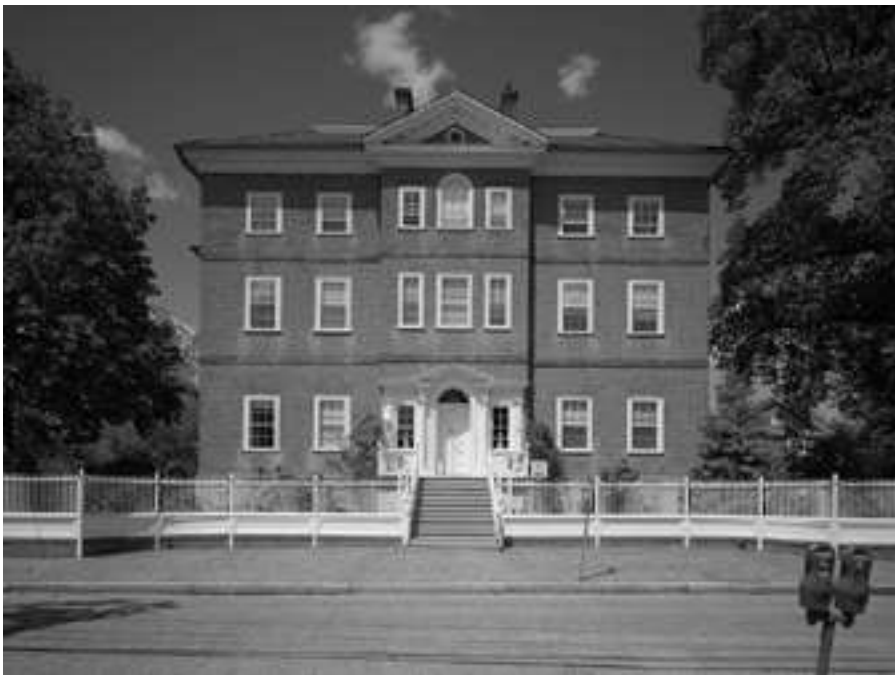
Chase-Lloyd House, Annapolis, Anne Arundel County, Maryland
