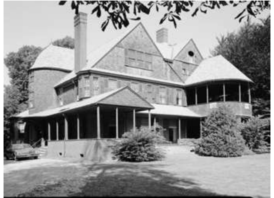
Isaac Bell House, Newport, Newport County, Rhode Island
