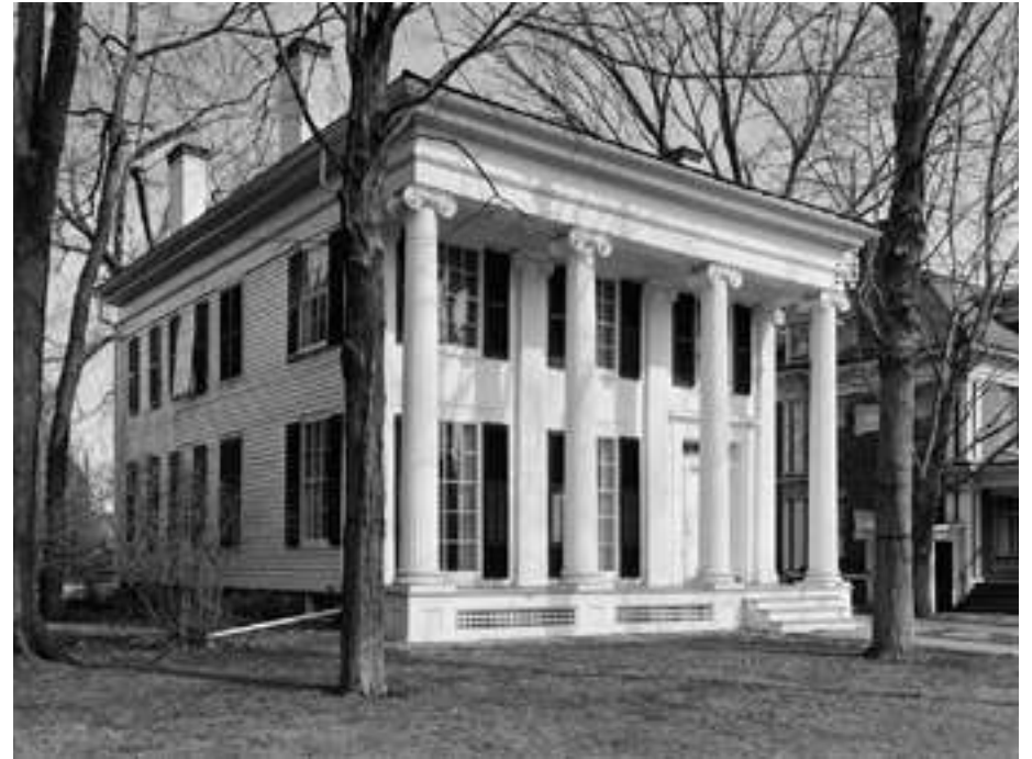
Joseph R. Jones House, Binghamton, Broome County, New York
