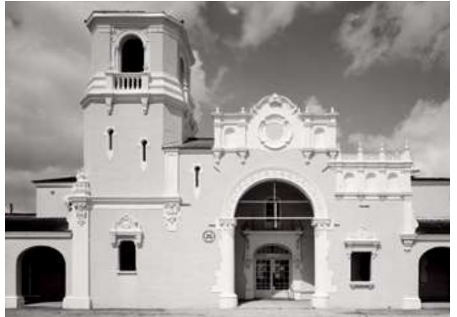
Seaboard Airline Railway Station, Palm Beach, Palm Beach County, Florida
