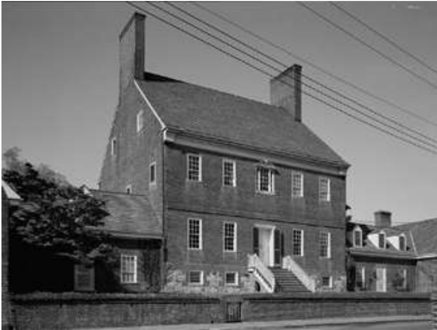
James Brice House, Annapolis, Anne Arundel County, Maryland
